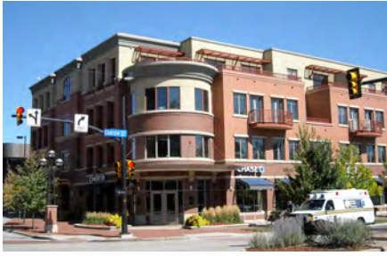
An entry to a mixed-use building should be easily identifiable and use a focal feature such as a rounded tower element.
