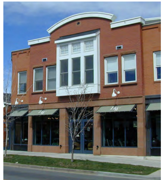
Articulate a building wall to create human scale components and express a sense of vertical and horizontal scale.
